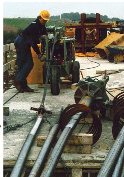
Hydraulic pushing machine on pump unit: Insertion into post-tensioning ducts using a flexible strand guide.
