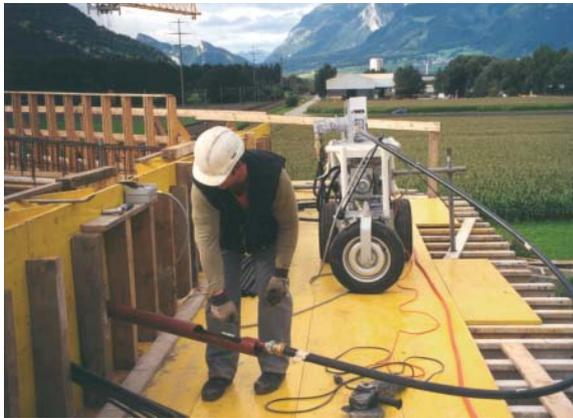
Because of this the machine is ideal for the manufacture of single-span beams, floors, tanks etc. The hydraulically driven pushing machine with six pairs of rollers is suitable for the insertion of strands of maximum lengths of 200 to 300 m and is therefore ideal for bridge building.
