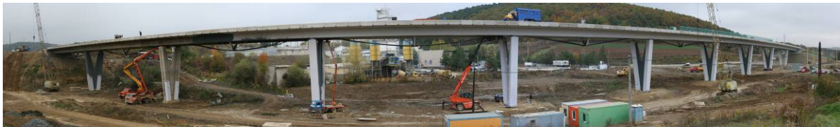
Fig. 1 Panoramic perspective of the whole bridge structure during the construction period
