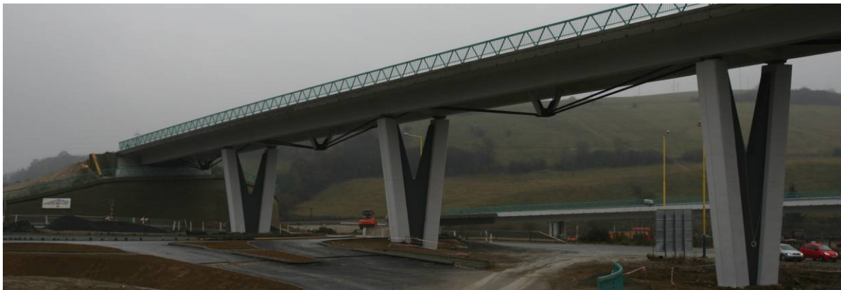
Fig. 2 Part of viaduct 215-00 during the construction period
